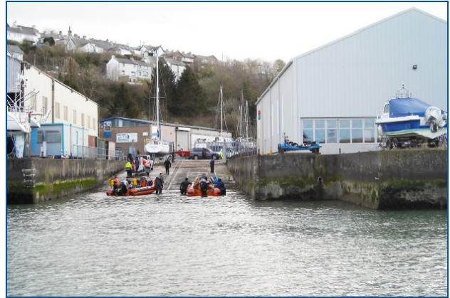
The Slipway at high-water
