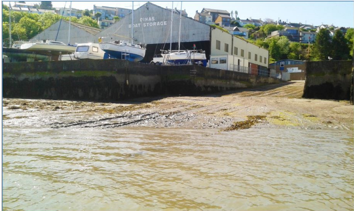
The slipway at low-water. Note the wheel-tracks in the mud.
